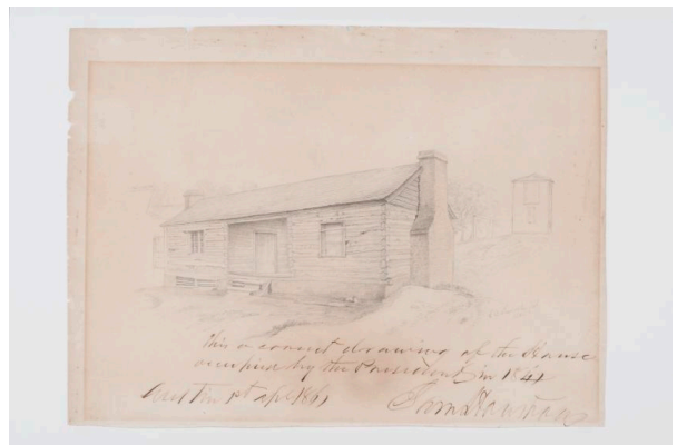
Window mat lifted
